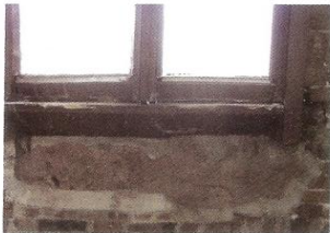
Bell Tower Interior
