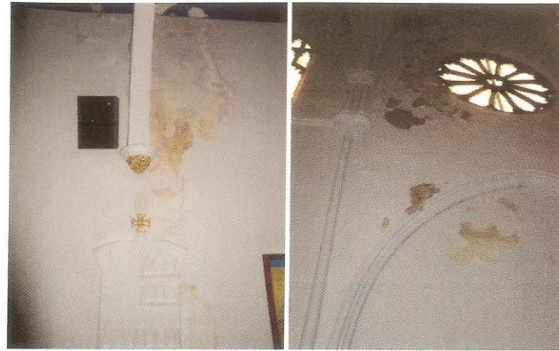
Damage to the interior wall surrounding Rose Window Debris from the ceiling/wall deterioration
